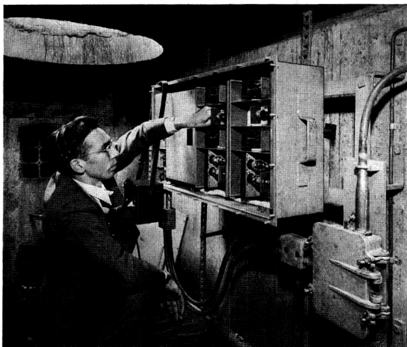
Fig. 5—Million-cycle repeater mounted in a manhole.
