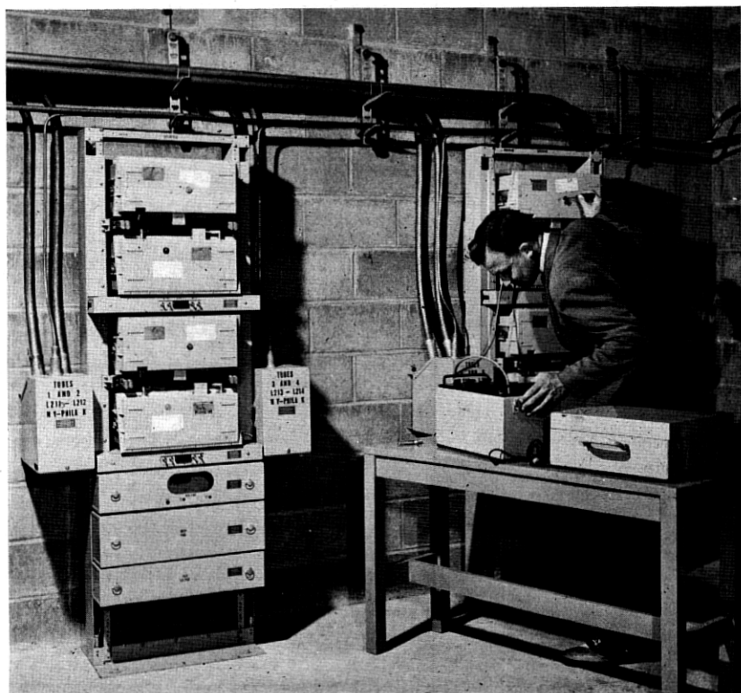
Fig. 23 — An engineer testing pilot transmission in an L3 repeater hut.
