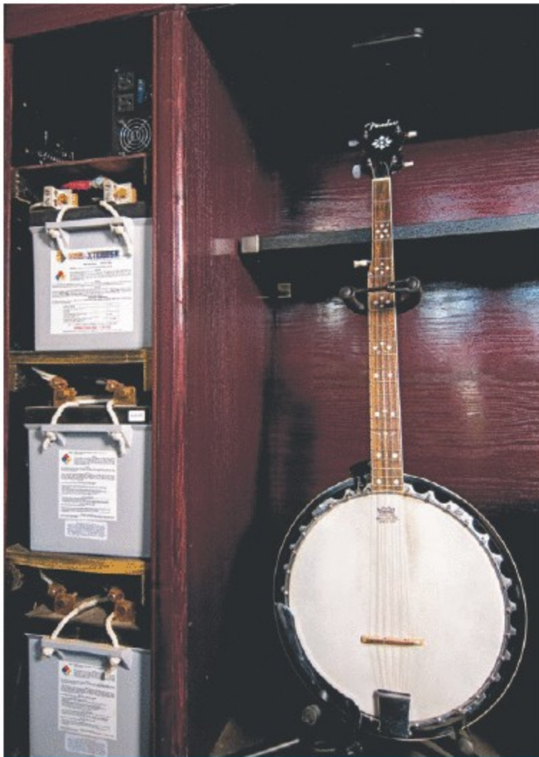
ABOVE: AGM battery bank stores solar power for the studio, while a banjo provides inspiration to visiting cowboy poets. RIGHT: Power center contains all the equipment needed for off-grid electrical generation.
